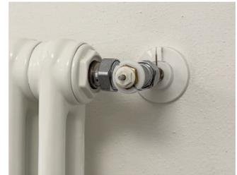
2) Install the adapter if necessary. Contact your plumber to find the correct adapter. If necessary for installation, remove the plastic cylinder on the bottom of the TRV+AA by sliding it outwards.
