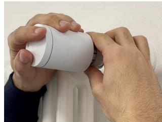
5) Install the TRV+AA smart thermostatic valve by screwing the ring nut onto the adapter thread (or valve thread) in a clockwise direction.
