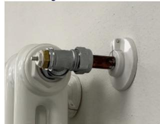
1) Remove the old manual thermostatic valve from the radiator.
